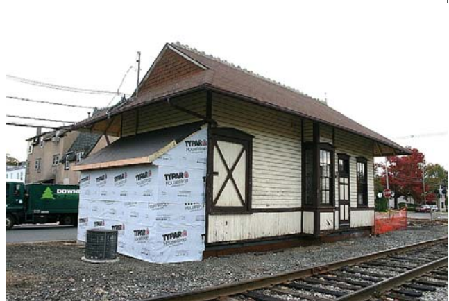
The addition framing completed
