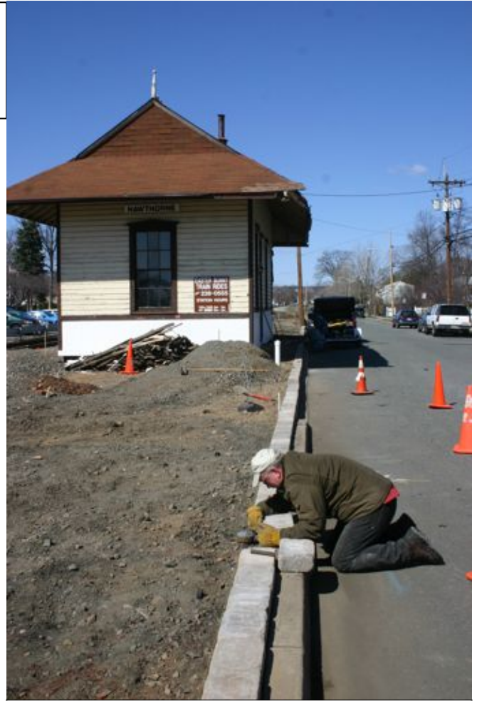
VRA President KC Smith works on the new curbing along Royal Avenue.
