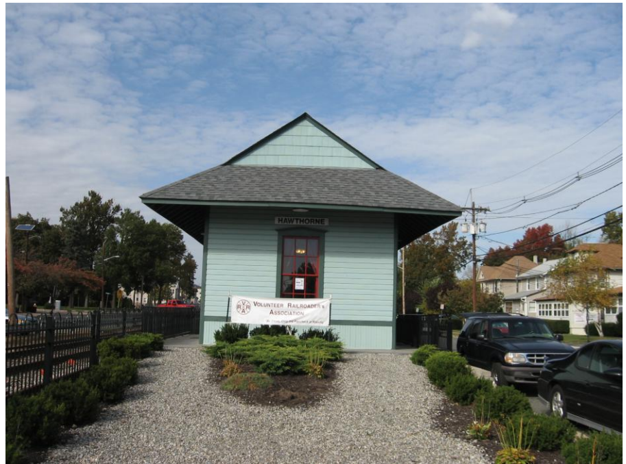
The finished ends on the east end of the station.
