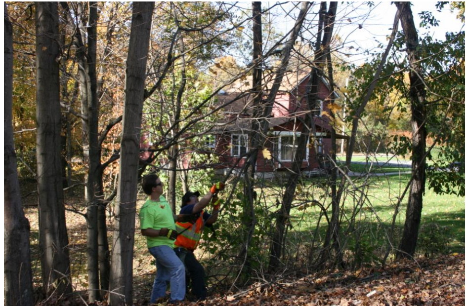
Justin Kerstner and Matt Phalon removing tree limbs fouling the main near MP 15 near Toys R Us. "Maintaining the way."
